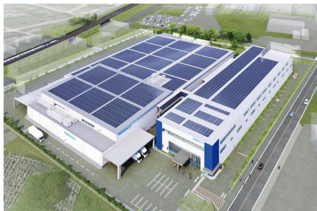
Illustrative image of the new building
