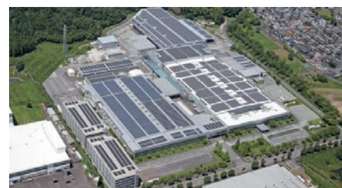
Solar panels installed at the Tsu Plant
