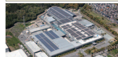
Solar panels installed at the Tsu Plant
