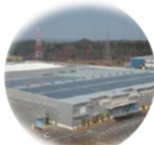
2016 Tsu Plant 500kw
