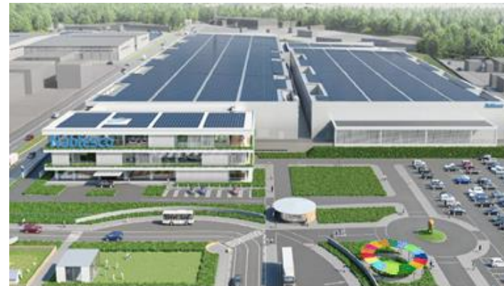
Onsite solar panels
