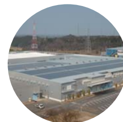
Solar panels at Tsu plant
