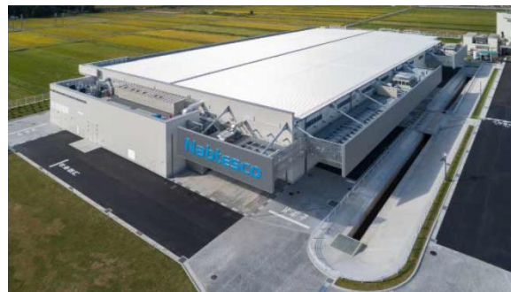
Building for actuators (Total floor area: 8,263 m 2 )
