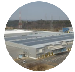
Solar panels at Tsu plant
