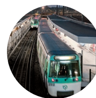
GILGEN platform doors (bijou(R)): Paris Metro Lines 1 and 13
