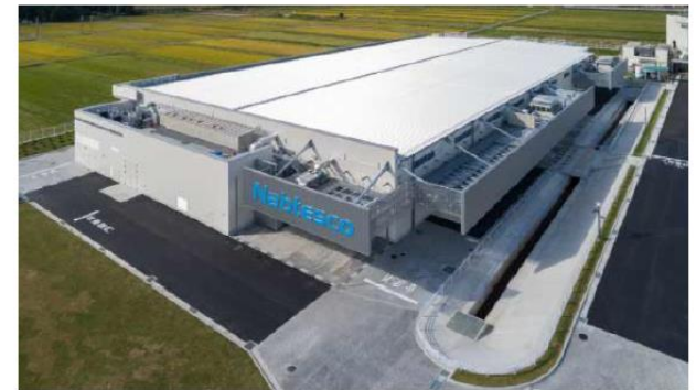
Building for actuators (Total floor area: 8,263 m 2 )
