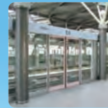
Platform screen doors
