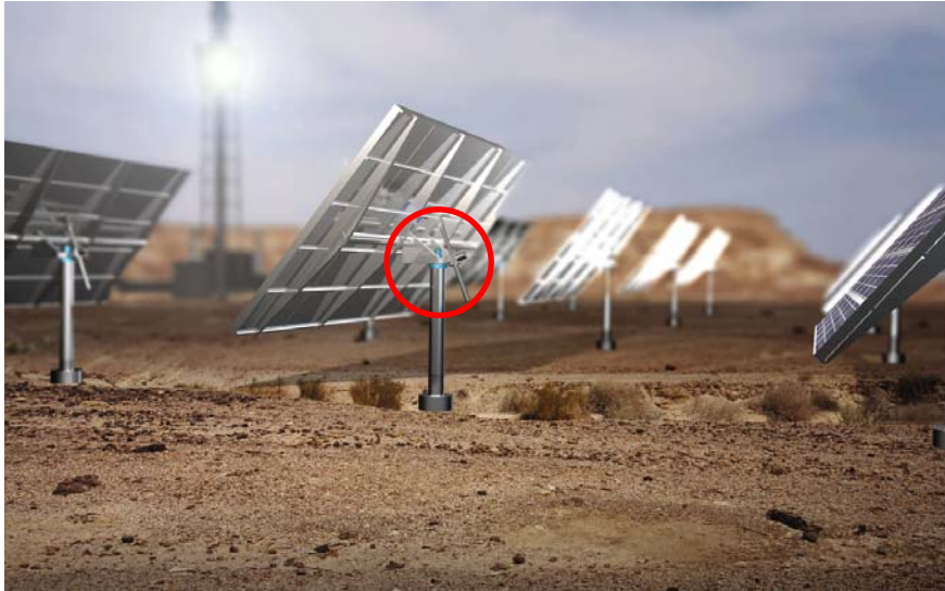
*The solar tracking equipment(Azimuth drive) on the rear of a heliostat (image)
