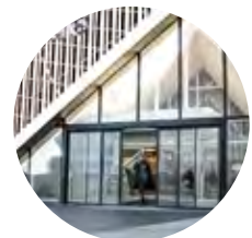
GILGEN doors: Westside Shopping and Leisure Centre in Switzerland
