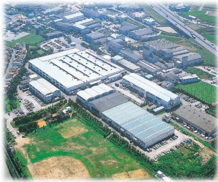
Seishin Factory (Nishi-ku, Kobe City, Hyogo Prefecture) / Marine Company Mother Factory
